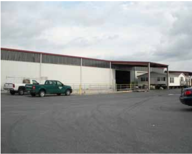
Stock Building Supply – Millwork Building On-Site
