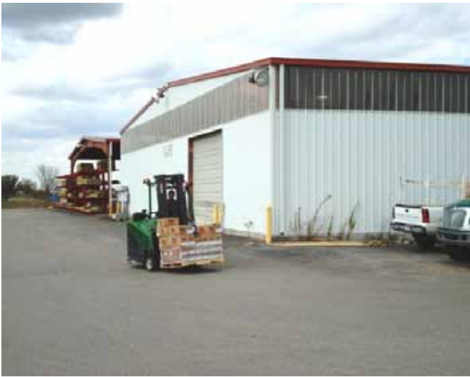
Stock Building Supply – Millwork Building On-Site
