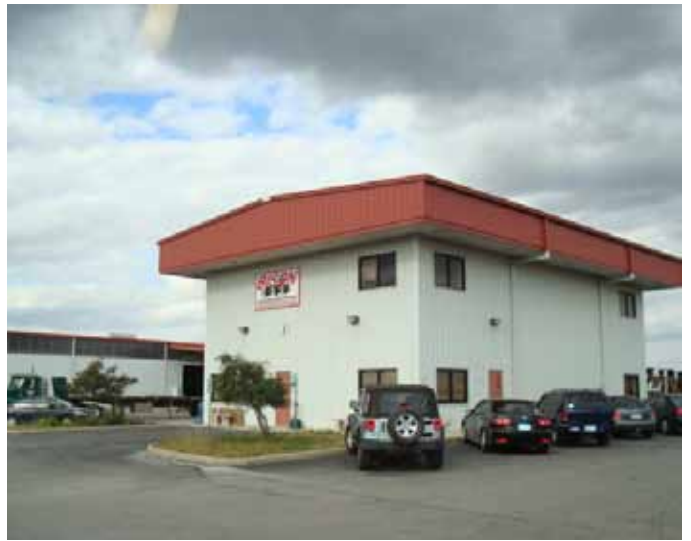
Stock Building Supply Office On-Site
