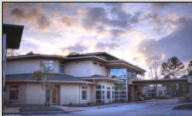
Main Building Side View
