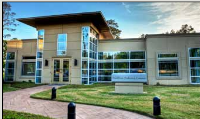
Office Building Two Showing "Prairie Style" Reflective Glass
