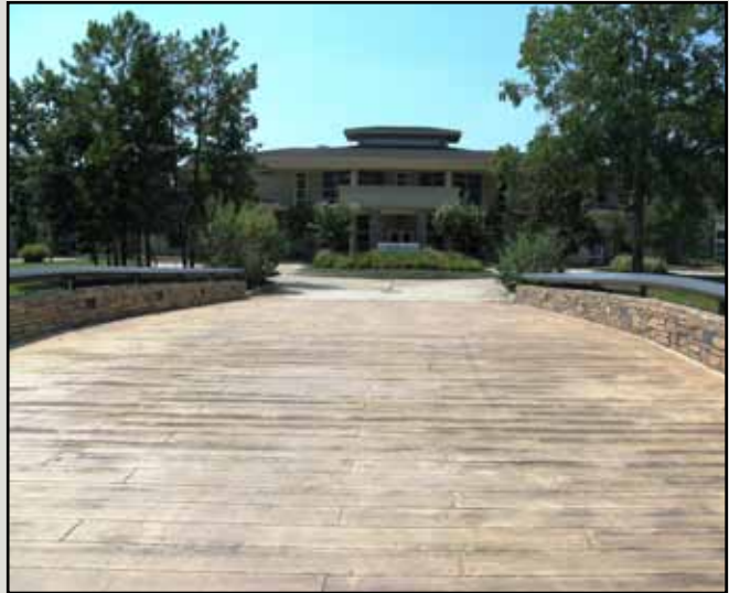
Lake Bridge View of Main Office Building
